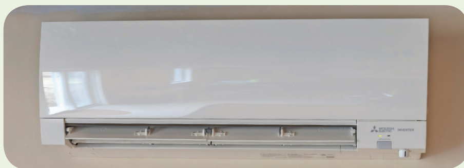
A wall-mounted indoor air-handler unit in the basement of the Rileys' home in Peterborough.
