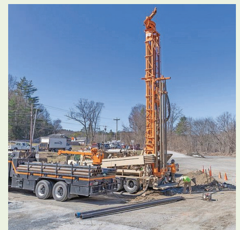
Cushing and Sons Well Drilling at work on geothermal wells for Sugar River Storage in Claremont. (Aaron Lipsky photo)
