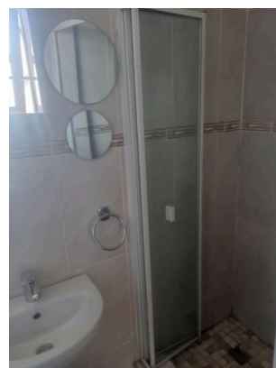
LEFT: A photograph of the “accessible step-free shower” at one establishment, which clearly has a step.
