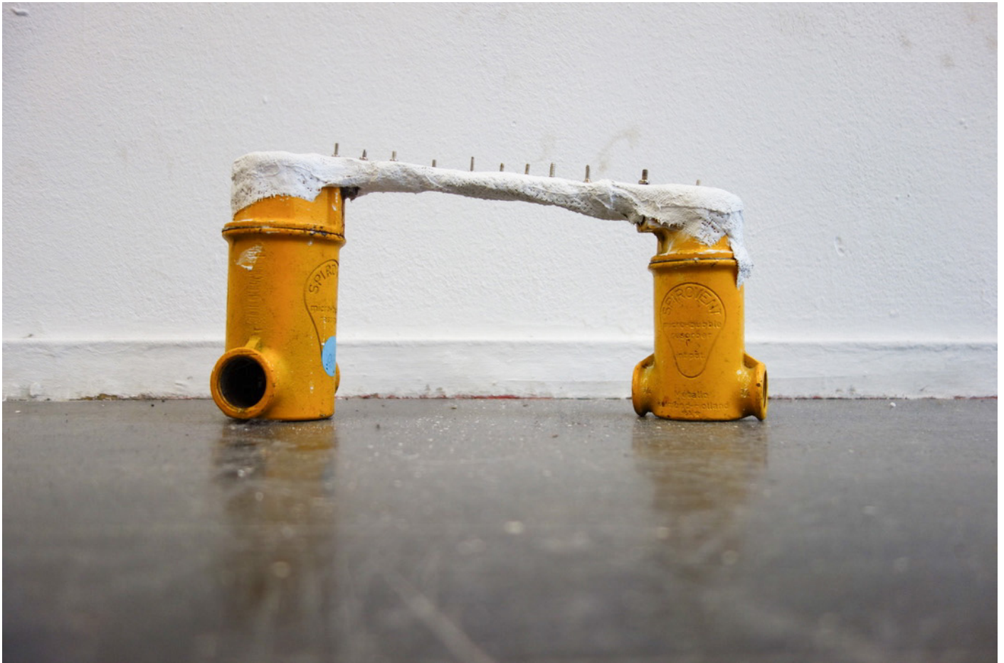
Spirovent connection (Overview photo)
