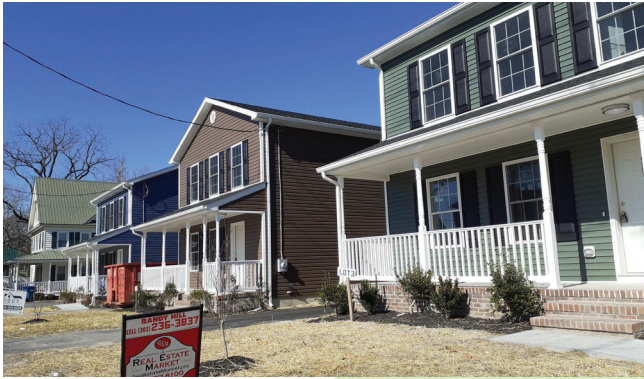
Milford Housing Renewal in Milford, DE
